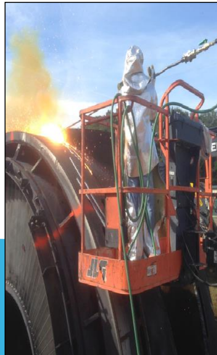
Demolition of LP Turbine system for Robinson Nuclear Plant
